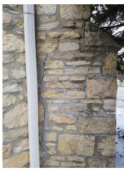
Last Friday E&H Restorations was here to install some helical piers under a crumbling buttress but determined that the foundation of the church had deteriorated to the point that the fix was not possible - they are currently trying to come up with an alternative, and definitely more expensive repair. They did say that the building was still structurally sound, but that repairs should be done sooner than later.
